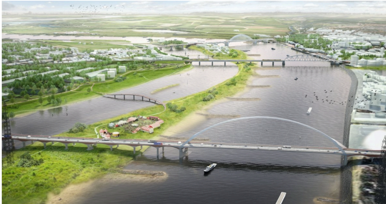
The Dutch city of Nijmegen is building a flood-control channel for the River Waal (left). In the process, it is also creating an island for recreation as well as prime property that can be developed into a new heart of the city. (Room for the River Waal)
